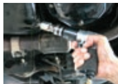
DRILLING DRAIN HOLE
