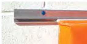
"C" channel mounting with walt strip.
